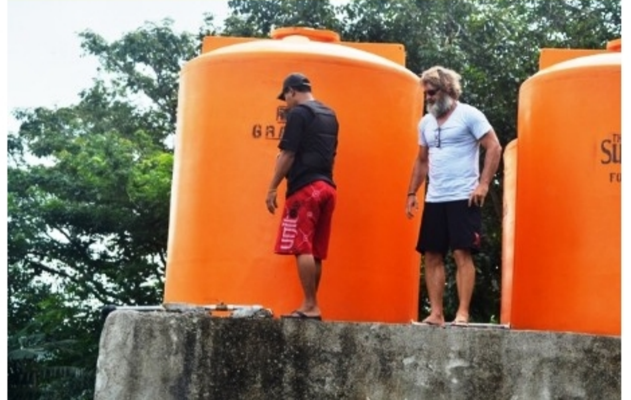
Above: Dr Stephen Nolan inspecting the main water station in Patiala Dete with water team leader (Rudy Weru).
