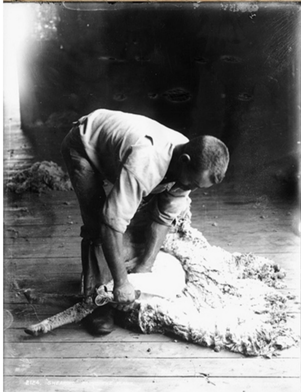
Above; 'Shearing around the flank'
