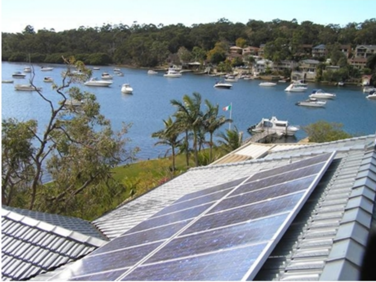
Above: Northern Beaches installed domestic system
