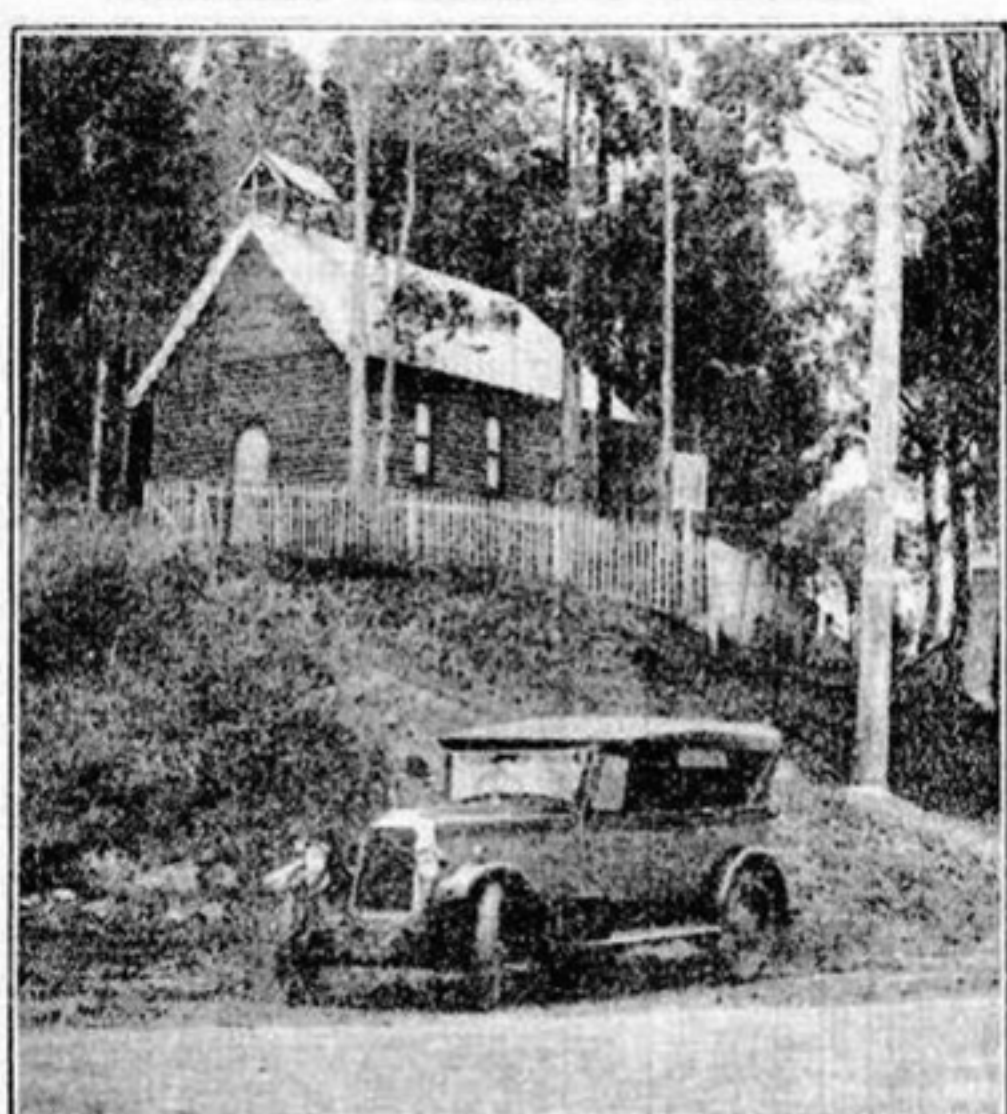
A proposal to demolish the old Methodist Church at Church Point, Pittwater, is criticised on the score that it should be preserved on account of its historic associations.
